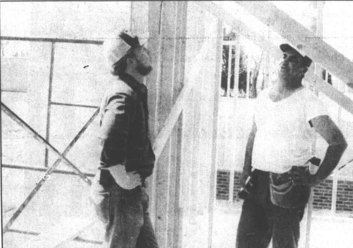
Above Willie Whitehead and Aubrey Ownly, Jr., the Perquimans County building inspector examine a house currently under construction in the New Hope area of the county. This house is just one of many currently under construction which must be inspected by Ownley before they are completed.
