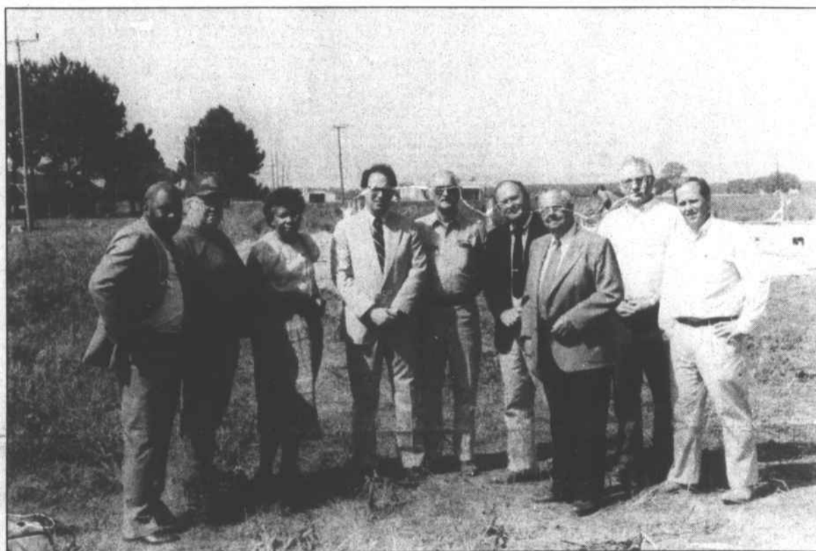
Cement has been poured for Pala Engineering, a new business expected to open in Hertford this summer. Community and business leaders came out to welcome Frank Pala to the area.
