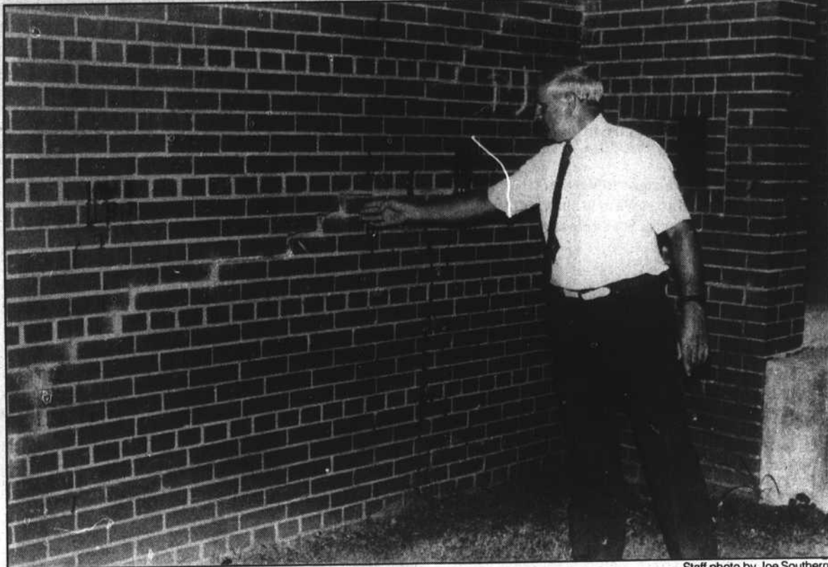
Perquimans County Board of Education member Wayne Howell points to a large crack in an outer wall at the vocational education building at Perquimans High School. The wall is separating from the building and is slowly falling away.
