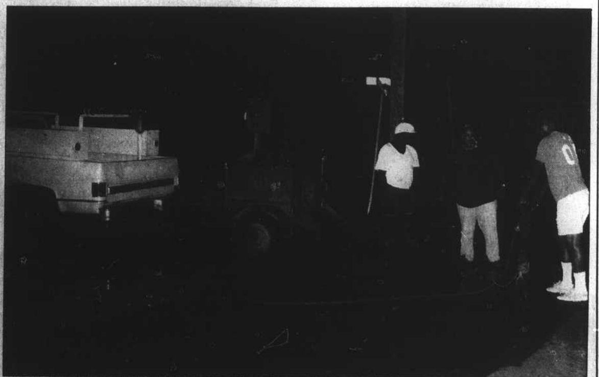
A leaking water pipe in front of Cannon's Cleaners on Grubb Street brought town maintenance crews out around 8:30 Monday night. Hertford town manager Bill Cox said it took about two hours to fix the leak. Cox said the town couldn't afford to lose water
