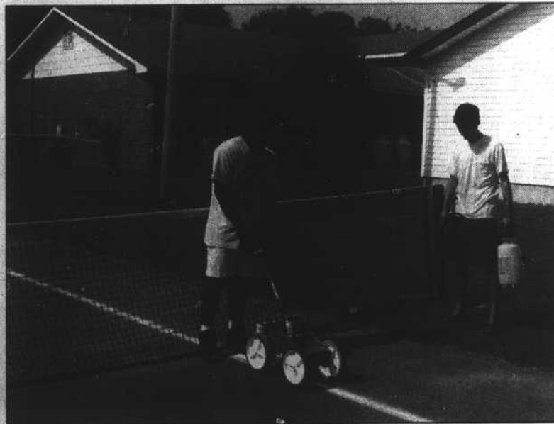
Jermaine McClenney fixes the striping on the tennis courts while Ben Waters sprays to control weeds around it. The youth are working for the recreation department this summer under the JTPA program. JTPA is a federal program designed to provide on-the-job training and summer employment for qualifying youth. (Photo by Susan Harris)
