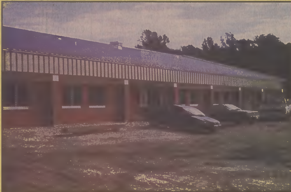
Construction is on schedule at the new Central School in Winfall, according to supervisors with M.B. Kahn Construction Company. Kahn anticipates that students and teachers will be able to move into the new facility sometime in January or February.
