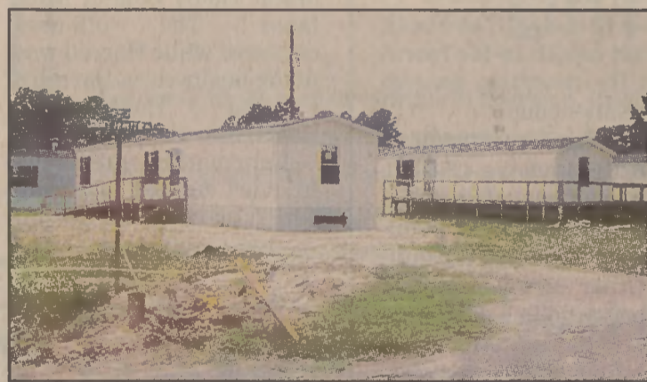
Four mobile units sit in what was formerly a parking area between the high school and the schools' central office.
