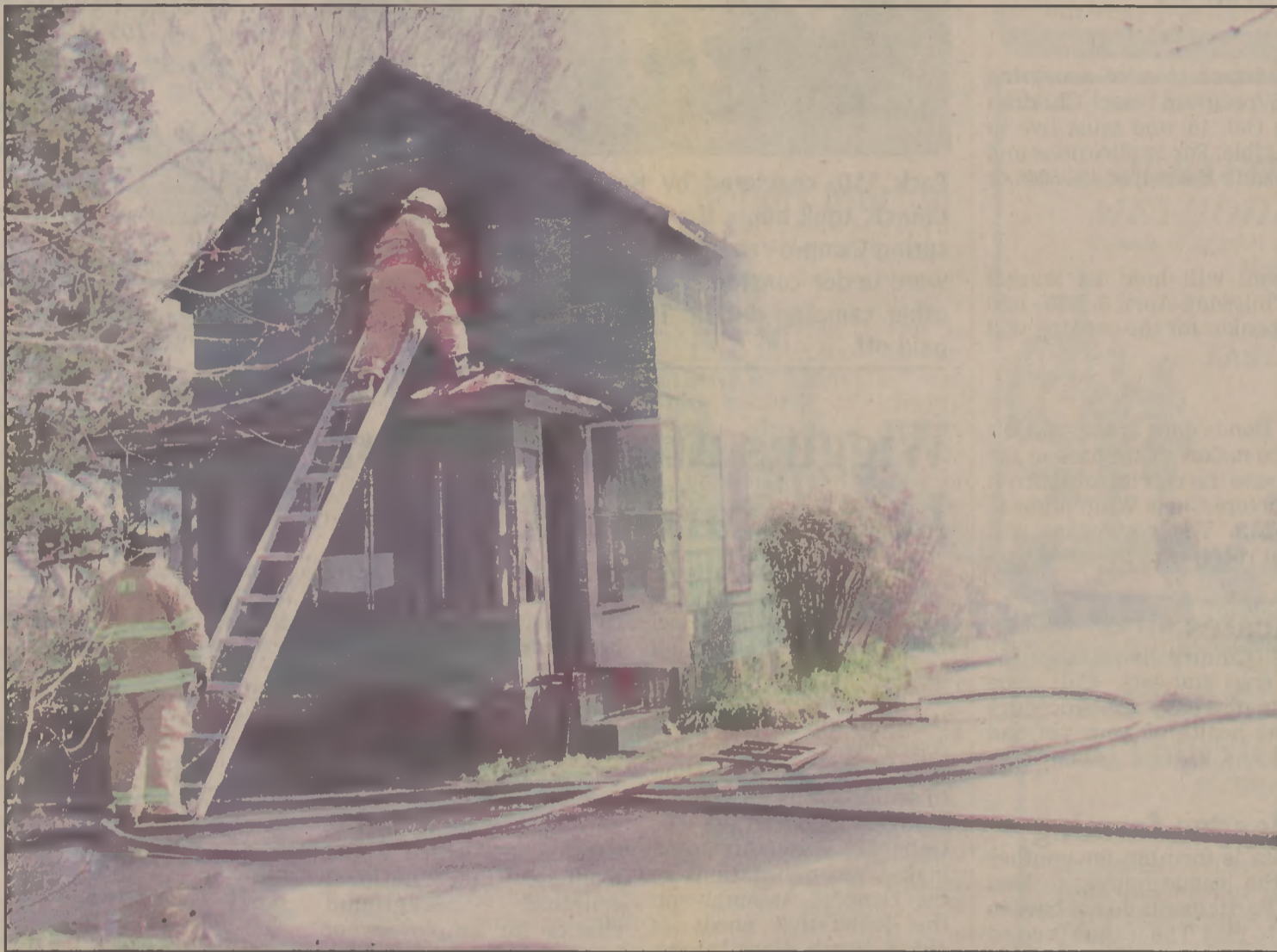
Winfall and Hertford firefighters battle a house fire on Loomis Street in Winfall Monday morning. The initial investigation suggests the fire began at the water heater. The home appears to be a total loss.
