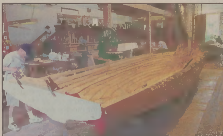
Workmen at the North Carolina Maritime Museum in Beaufort build the periauger to be christened June 19.
