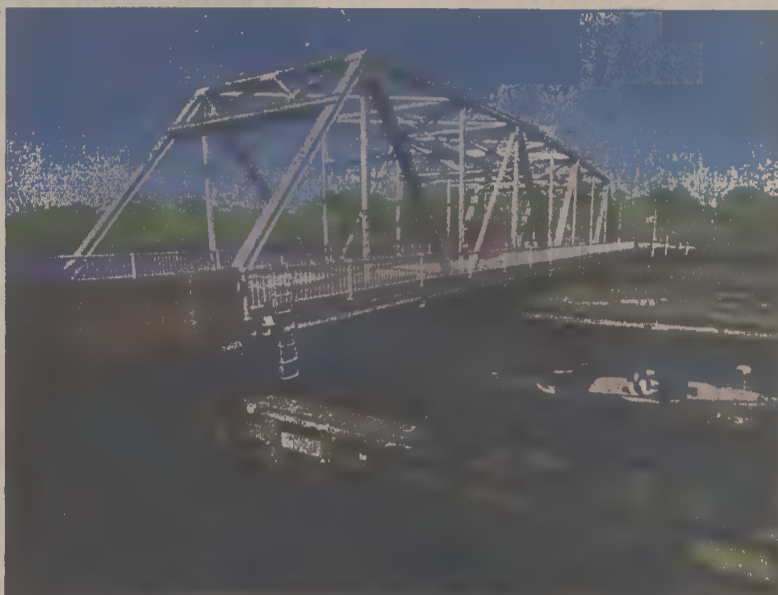
The S-Bridge in Hertford has a swing-span that allows taller boat traffic in and out of the riverfront near the town. A group of residents wants to save the bridge, which is scheduled to be replaced.
