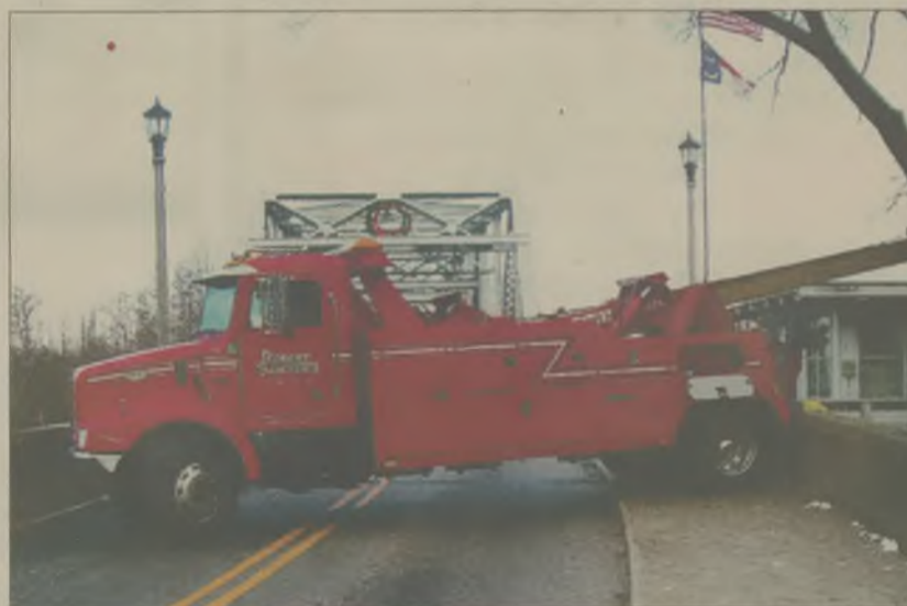
A boom truck blocks the S-bridge while workers raise the pickup truck from the river.
