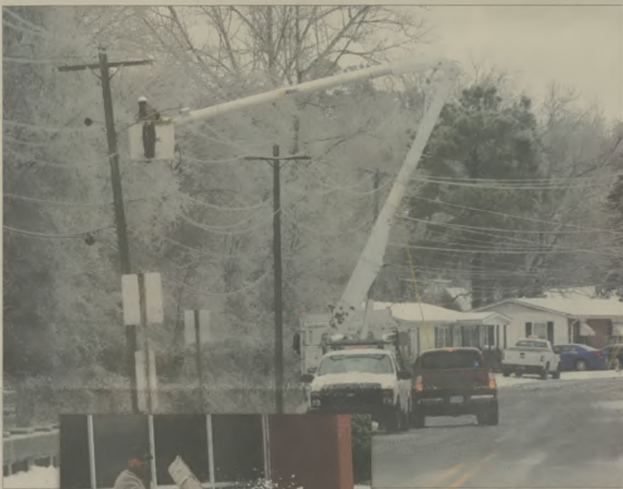
A lineman (above) from the Town of Hertford clears away limbs near power lines on Church Street on Feb. 17 after an ice storm.
