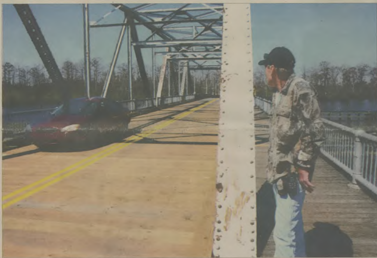
Bill Cartwright, one of the bridge tenders on Hertford's S-Bridge, watches a car drive across the bridge Friday afternoon. The bridge underwent three months worth of repairs to make it lighter in the hopes of extending the life of the span by a few years.
