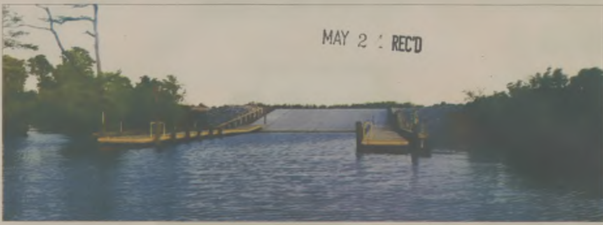
A view of the new Hertford boat ramp from the water.
