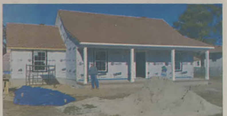
PHOTO COURTESY CHOWAN-PERQUIMANS HABITAT FOR HUMANITY
