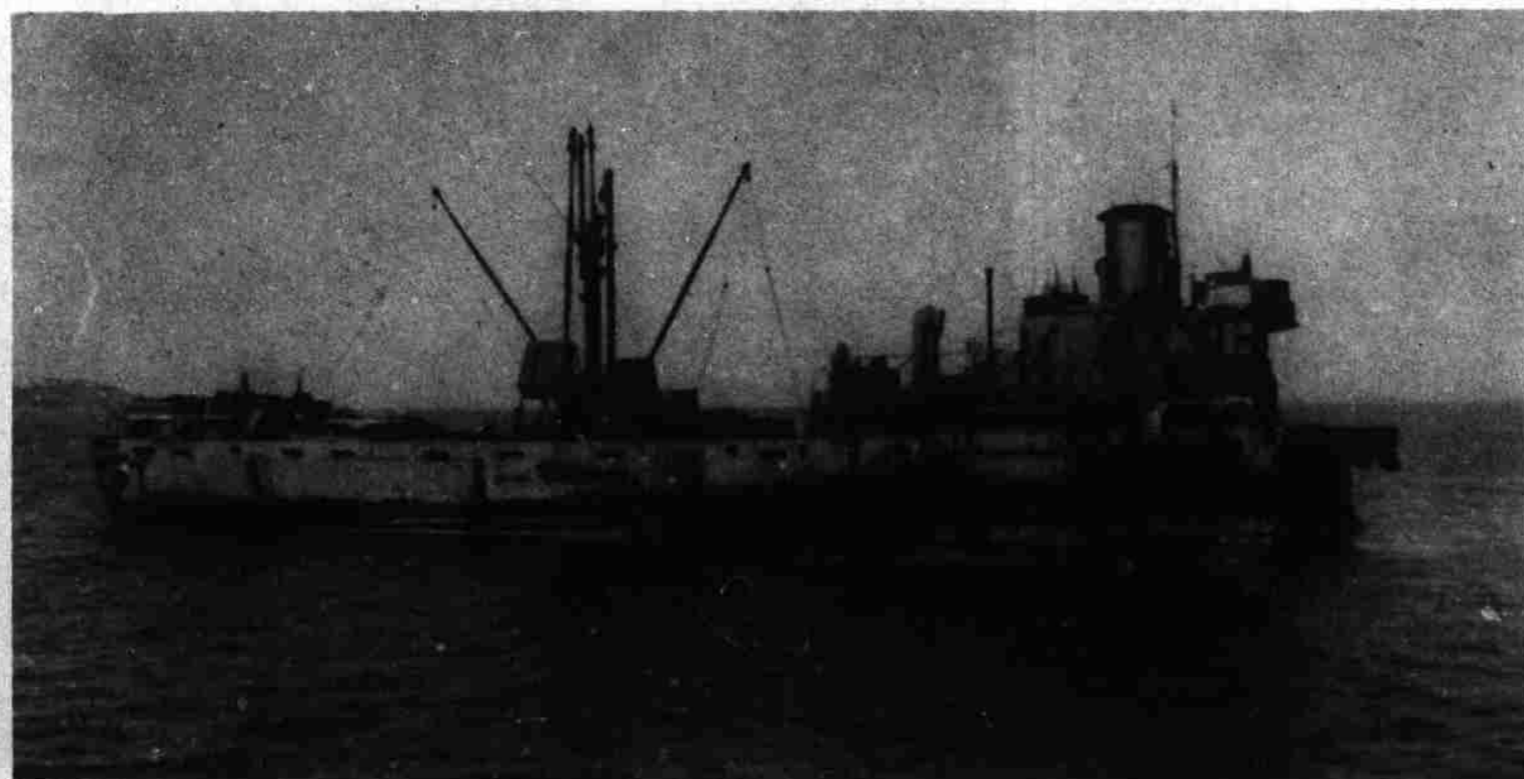
When the S. S. Virginia Dare, our hull No. 3, struck a mine in the bay of Tunis early in March of 1944, the powerful explosion blew the bow of the ship off just forward of bulkhead No. 68. The vessel was abandoned but the aft section was later salvaged by a tug. The above picture of this section was sent to The Shipbuilder by Leslie Walker, former member of the Hull staff now stationed at the Sixth Port headquarters at Marseille, France. The S. S. Virginia Dare was launched Feb. 2, 1942, under the sponsorship of Mrs. Elwood Inge, and was delivered to the Maritime commission the following March 27.
