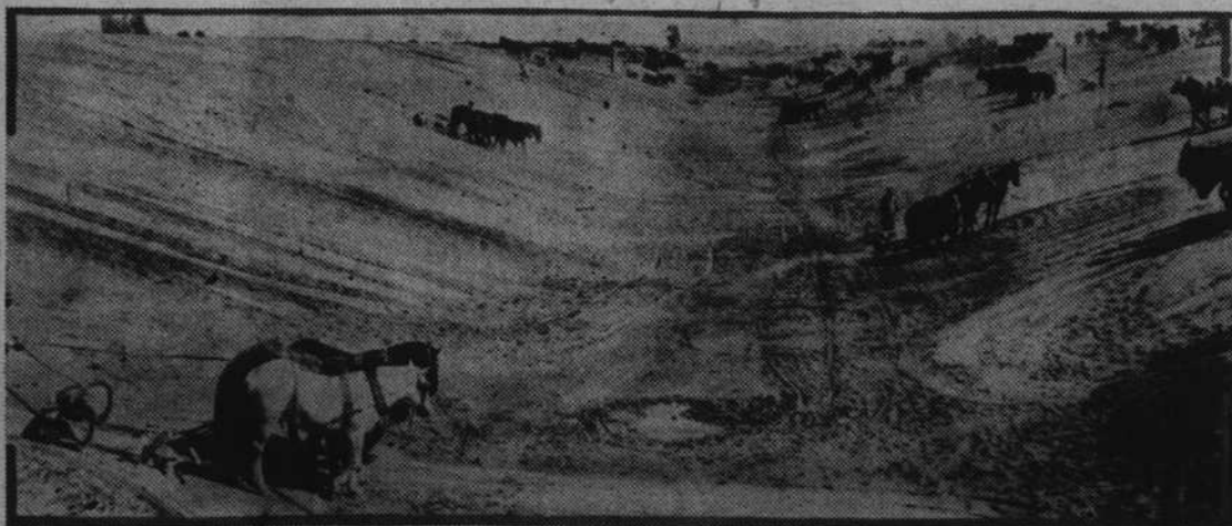
One hundred four-horse teams are here busy on one section of the All-American canal which will replace the main now serving California's Imperial valley. The new canal will have a width of 232 feet, a depth of 21 feet and will carry the water of the Colorado river 89 miles across the valley for irrigation purposes. The men and teams shown in the photograph above have moved more than 1,000,000 yards of earth with their Fresno scrapers.
