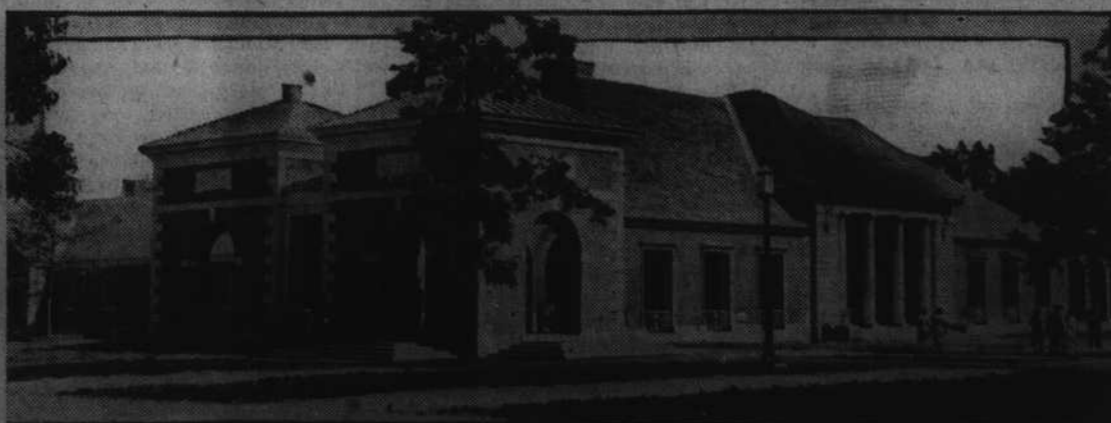
Gov. Herbert H. Lehman of New York dedicated this new $10,000,000 spa at Saratoga Springs, known as the Roosevelt Bath building. He described it as "another unique agency added to an already incomparable public health service."
