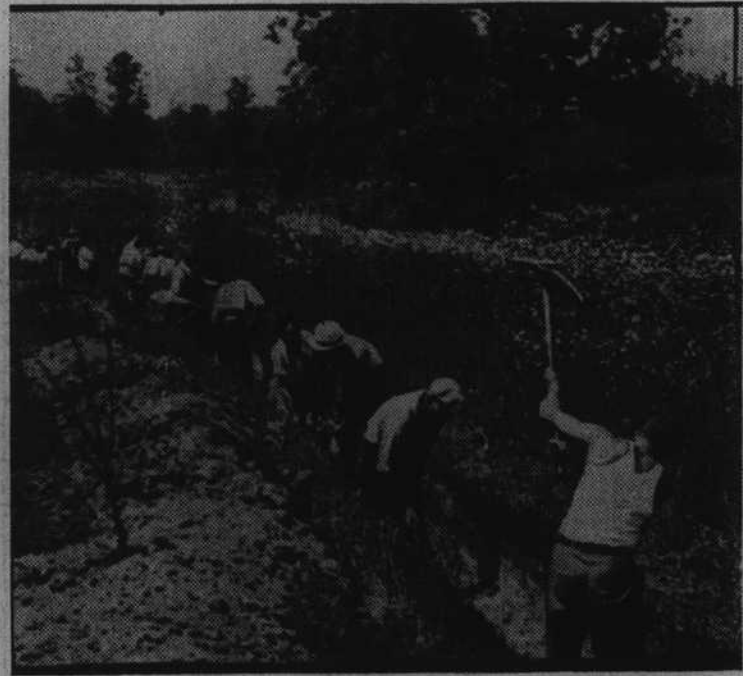
Workers are shown digging a water-line ditch, as work started on the housing project at Hightstown, N. J., where 200 subsistence homes are being erected on a 1,270 acre plot by the Federal Housing Administration.
