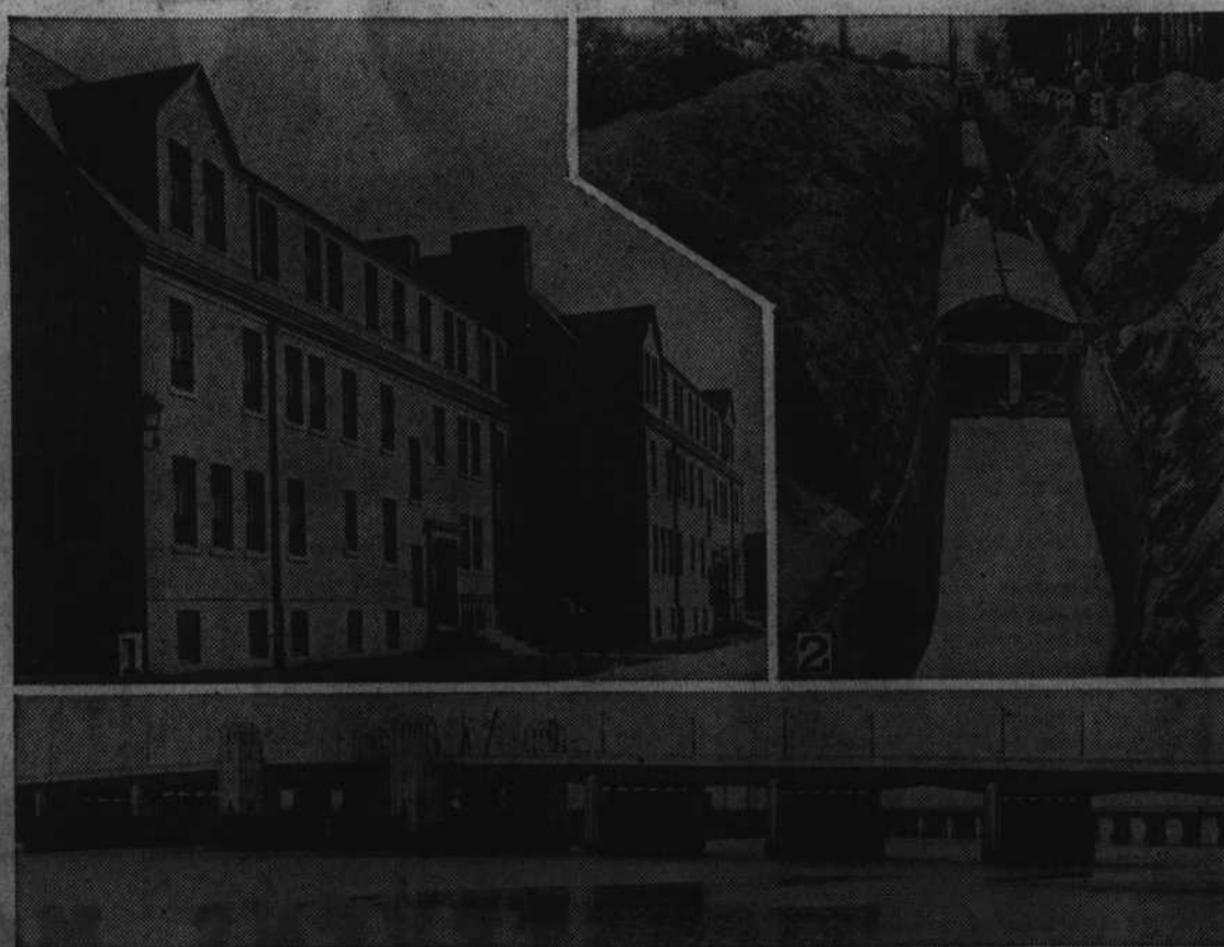
Here are three examples of the many and varied projects that have been made possible by allotments of funds from the Public Works administration: 1—New barless state prison colony at Norfolk, Mass., which received $763,000. 2—Storm drains in the orange country of California, being constructed with PWA money. 3—The new Point of Pines bridge carrying New England resort traffic from Lynn to Revere, Mass.
