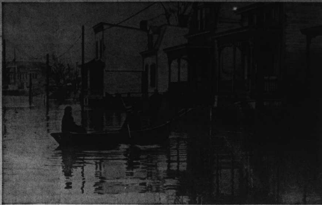
Police boat shown removing a water-imprisoned Cincinnati resident as flood waters following torrential rains swept the Ohio valley, inundating rural and city lands, causing deaths and untold suffering, as thousands of persons were forced to vacate homes and property, estimated at many millions of dollars, was destroyed.
