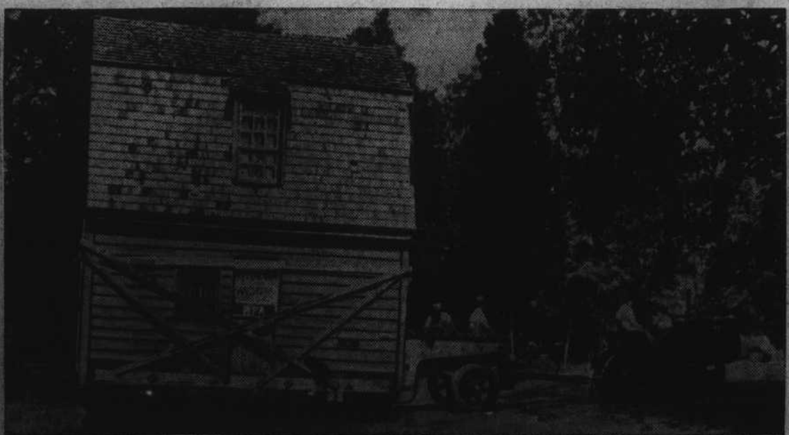
The humble cottage in which Andrew Johnson, who succeeded Abraham Lincoln to the presidency, was born, is loaded on a truck at Raleigh, N. C., and moved by WPA workers to its fourth site in its search for a permanent location. Originally the home stood near the state capitol, then it was moved to a location on East Caharris street and thence to Allen Park.
