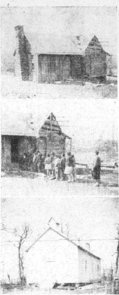
Bottom picture—The Cherry Lane Colored school building which has been repaired and painted by NYA boys.
