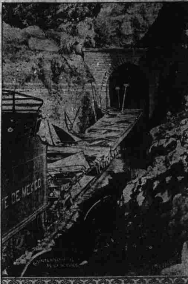
This is the south entrance of the Cumbre tunnel which Castillo, the Mexican bandit, set afire, causing the death of a number of men. In the photograph an engine is seen drawing out the wreckage of the train that ran into the blazing tunnel.
