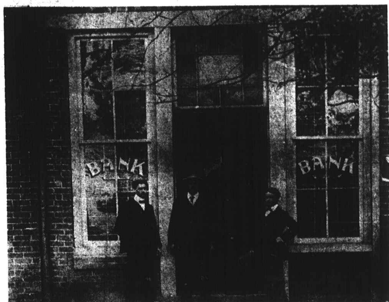
SCENE IN FRONT OF OLD BANK SHORTLY AFTER TURN OF CENTURY—Shown above is a picture of the First National Bank, as it appeared shortly after it was chartered. In the picture, left to right, are Dave H. Rudisill, now of Cherryville, the late W. F. Fulton, Kings Mountain merchant, and R. L. Mauney, at that time cashier and now a director of the bank.
