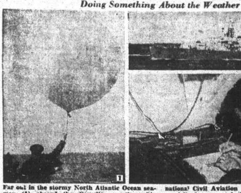
Far out in the stormy North Atlantic Ocean sea-men (1) aboard the Canadian weather ship H.M.C.S. St. Stephen, prepare to release a radio-equipped balloon which will radio back reports on weather conditions in the upper atmosphere. The St. Stephen (2) is one of 13 weather ships, supplied by eight countries and financed by 16, which make up a network arranged by the Inter-
