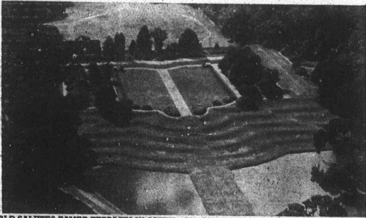
WORLD SALUTES FAMED TERRACES IN SOUTH —The 200th anniversary of the world-renowned terraces at Middleton Gardens in Charleston, S. C., is drawing international attention this year. The vast project—pictured here for the first time in an exclusive aerial view—was undertaken in 1741 under the supervision of Henry Middleton, President of the Continental Congress. His crew of 100 completed the Herculean task in 1750. The other famous gardens in Charleston are also preparing for their busiest season—Magnolia and Cypress Gardens, as well as Middleton, being open from Thanksgiving to May. Last year, Magnolia Gardens registered visitors from 26 foreign countries as well as from every state in the Union and from Alaska, Hawaii, and Puerto Rico.
