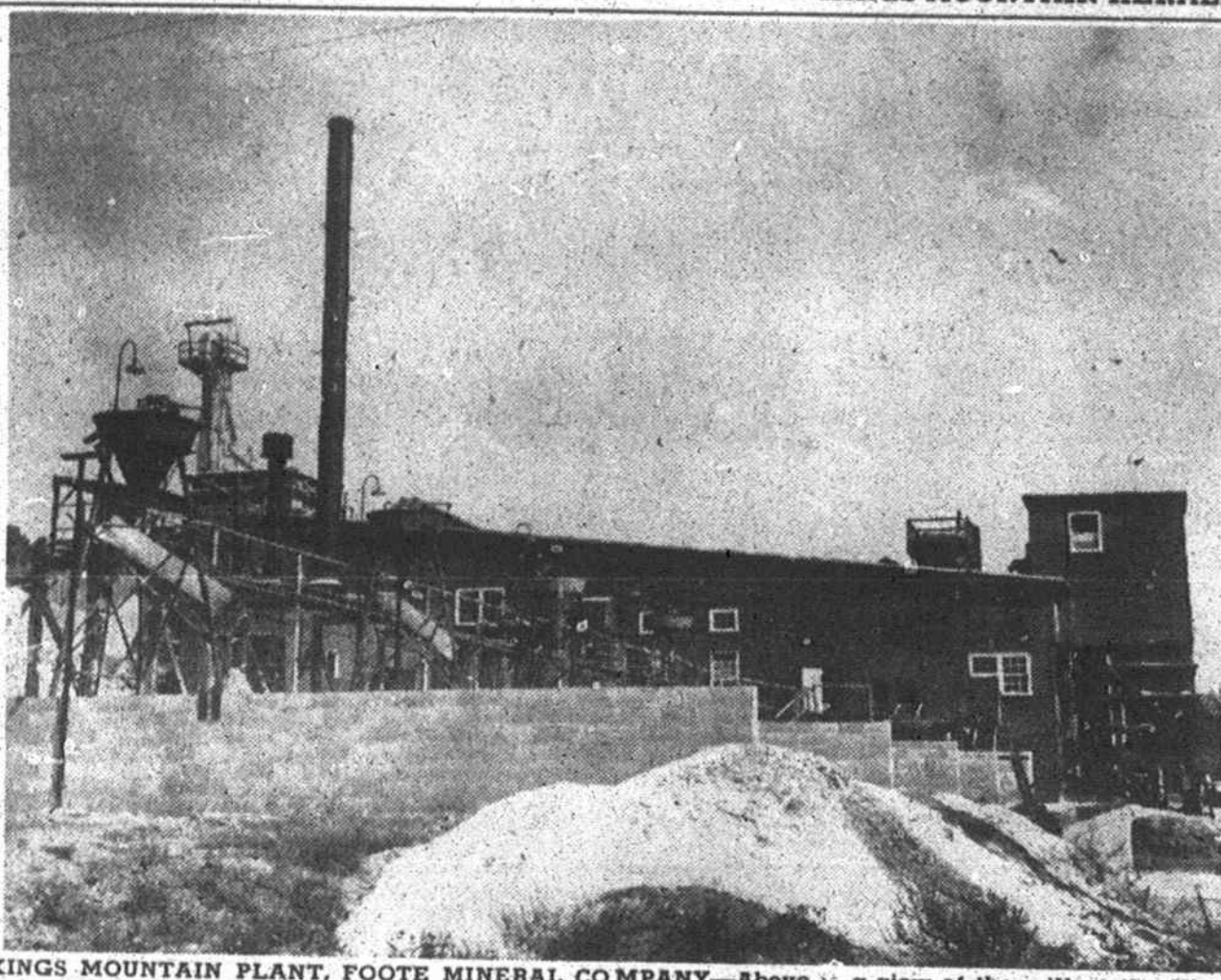
KINGS MOUNTAIN PLANT, FOOTE MINERAL COMPANY—Above is a view of the mill at the Kings Mountain plant of Foote Mineral Company. The picture was taken from the south side of the mill and shows drying bins in the foreground. The plant now has a capacity production of 360 tons per day on a 7-day, 24-hour schedule. (Photo by Carlisle Studio.)
