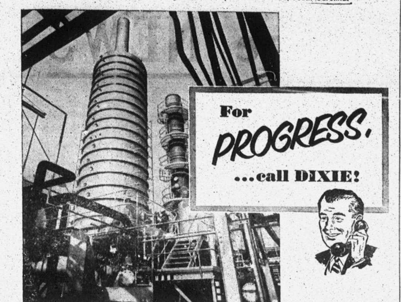
A good example of the growing industrialization and economic progress of the South is this new DuPont synthetic fiber plant at Camden, South Carolina.
