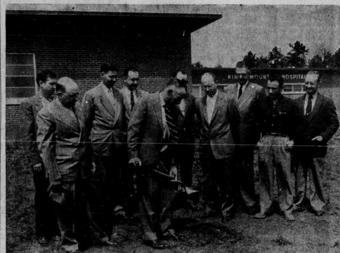
GROUND BROKEN FOR HOSPITAL ADDITION— County Commissioner Hazel B. Bumgardner dug the first shovelful of dirt Tuesday afternoon as ground was broken for the forthcoming 14-bed addition to Kings Mountain hospital. Others pictured, left to right, are Gene Clark, from the office of Ormand & Vaughan, the architects, Lewis Ho-
