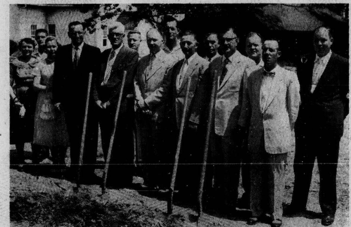
MACEDONIA GROUND-BREAKING — Macedonia Baptist church broke ground Sunday for a complete new church plant to be constructed on property adjacent to the present structure. Pictured are church officers, members and department heads who participated in the formal ceremonies. They are, left to right, Mrs. Roy Spake, Curtis Wright, Mrs. T. A. Lineberger, Rev. T. A. Lineberger, O. C. Kiser, Morris Timms, Henderson Her-
