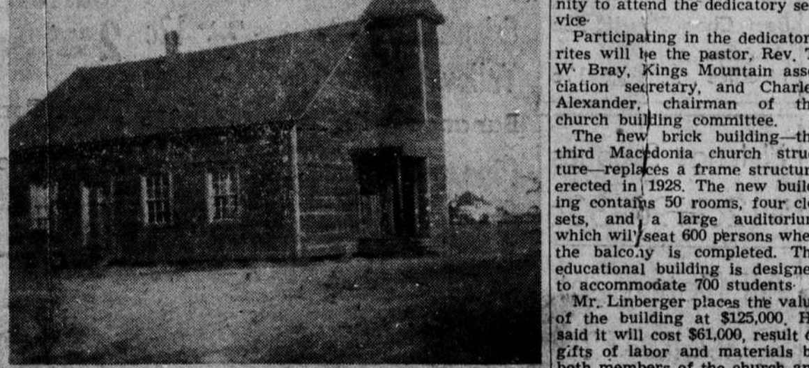
OLD MACEDONIA CHURCHES — Pictured above are the two buildings members of Macedonia Baptist church have used since its founding in October 1920. At top is the building the church will abandon Easter Sunday. It was erected in 1928 and will be razed to permit beautification of the grounds of the new church. Below is the first Macedonia Baptist church building, erected shortly after 1920, and first church erected by the Macedonia congregation.
