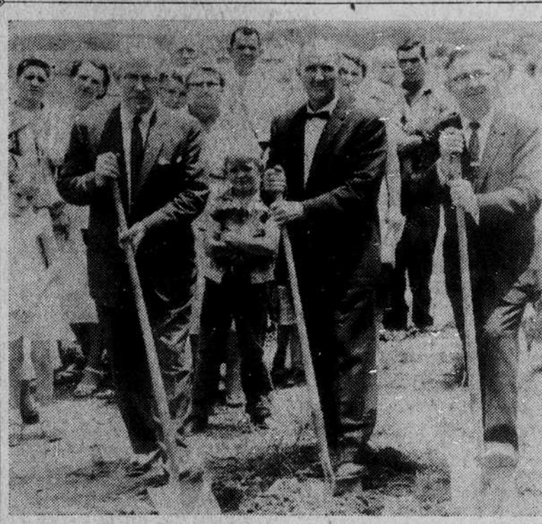
GROUND BREAKING CEREMONIES HELD — Penley's Chapel Methodist church on Cherryville road held groundbreaking exercises Sunday morning for a new church building. Dr. James G. Huggin, Jr., superintendent of the Gastonia district of the Methodist church, W. Leonard Huffstetler, Penley's lay minister, and Rev. W. C. Sides, Jr., pastor of the sponsoring Grace Methodist church, assisted in the ceremonies along with members of the official board and building committee. The new building will include a sanctuary and educational unit. Construction is under supervision of C. T. Bennett Construction company.
