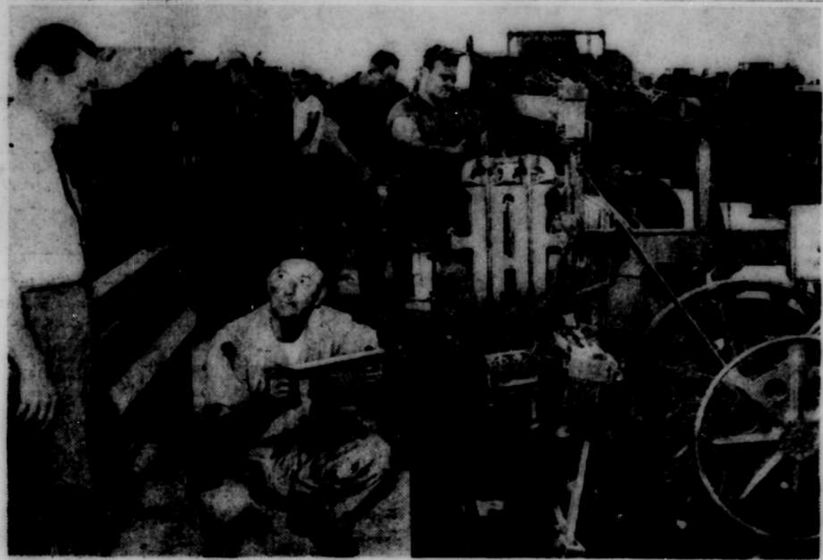
NEW TEXTILE FIRM INSTALLING MACHINERY — K. Mills, Inc., is busy installing looms at their new Marie street building. Pictured in foreground are Ralph Johnson, left, superintendent, and Tom Reynolds, overseer of machinery installation in background, left to right, are Donald Cobb, Richard Proctor, Paul Bridges, and Foley Cobb, Jr. Supt. Johnson said he would begin processing employment applications next week. The firm will manufacture upholstery fabrics.
