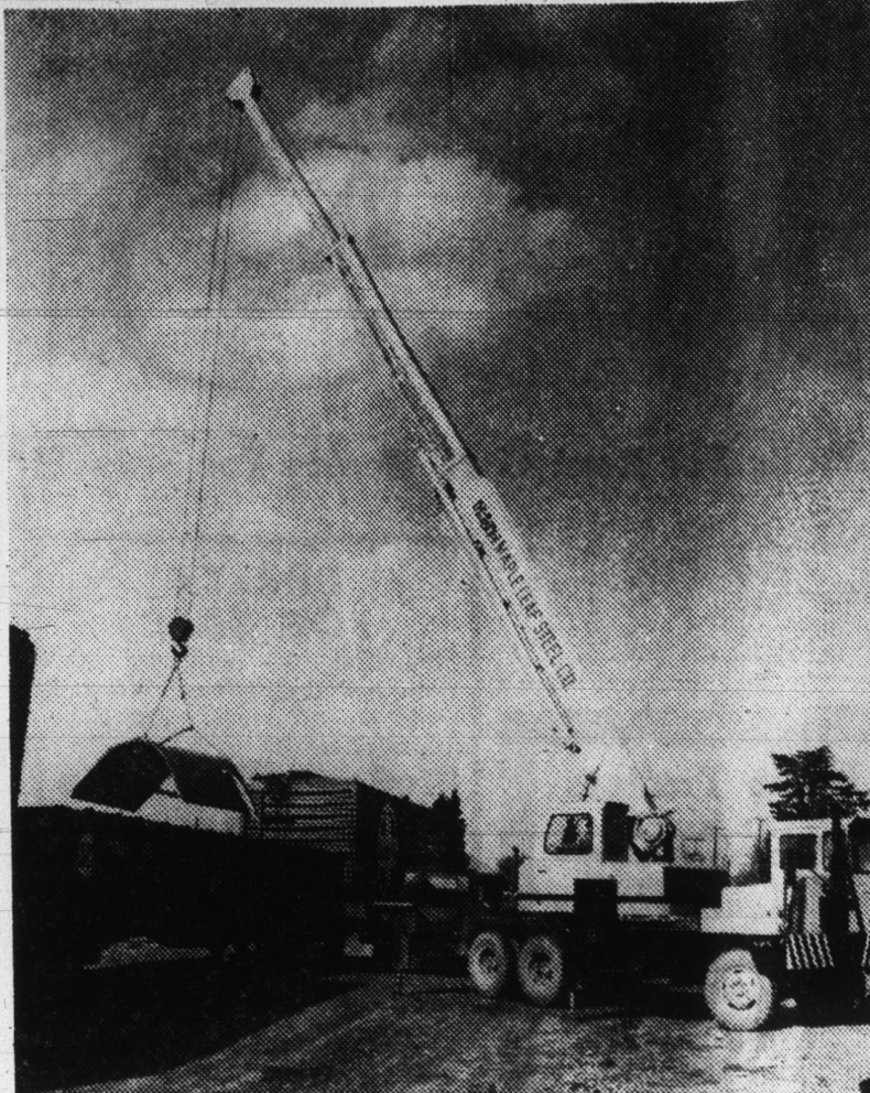
BIG CRANE ON THE JOB — Maple Leaf Steel Company, Inc., recently acquired a Grove 15-ton capacity crane, completely hydraulic, with an 82-foot boom.
