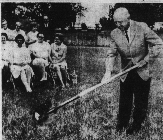
GROUND BREAKING — George W. Mauney, chairman of the board of trustees of Kings Mountain hospital, dug the first spadeful of earth as ground was broken Thursday for a $1,033,917 addition to Kings Mountain hospital. Mauney took a brand new shovel and dug into the grass of the front lawn where the two-story wing will be built, adding 35 beds to the facility with new operating rooms, labs, pharmacy and expanded x-ray facilities. Construction will begin Monday and the 23,000-square-foot east wing should be completed in 18 months. (Paul Lemmons Photo).
