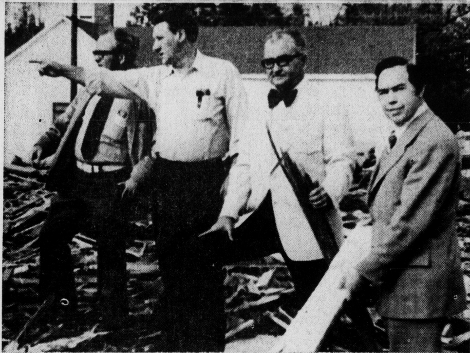
BEAUTIFICATION INSPECTORS — Norman King, second from right, and interested city employees look over a dwelling which was demolished on Wells Street last week as part of the annual Clean-Up, Paint-Up, Fix-Up campaign.
