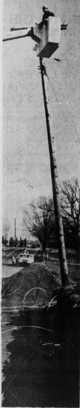
UP HIGH — Riding the cherry picker is a city employe preparing to remove this utility pole from the W. Gold St. right of way. The street is being widened to reduce bottle-neck traffic conditions in the central business district.
