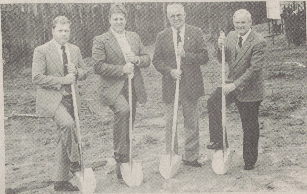
GROUND BREAKING - Ground was broken Saturday at the site of the new Eng School of Self Defense on North Piedmont Avenue. Left to right are Robert Walker, contractor; Robert Eng, owner; Mayor Kyle Smith, and Rev. Oscar Stalcup, pastor of Foursquare Gospel Church.
