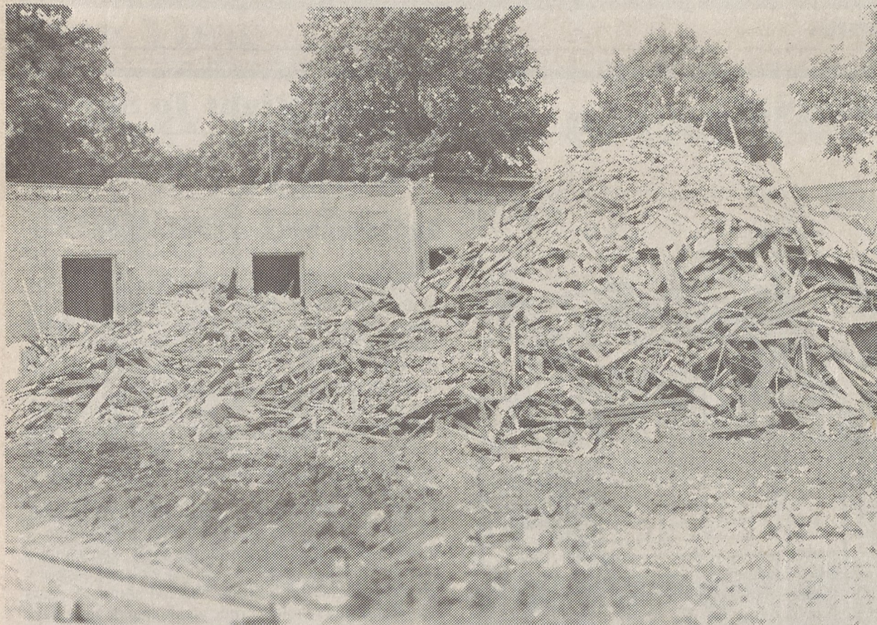
West School being torn down
