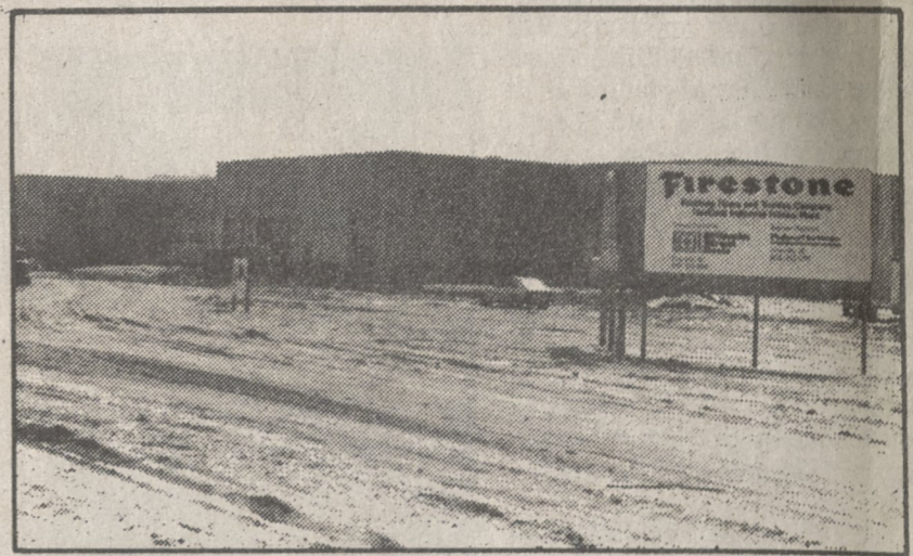
Firestone plant nearing completion
