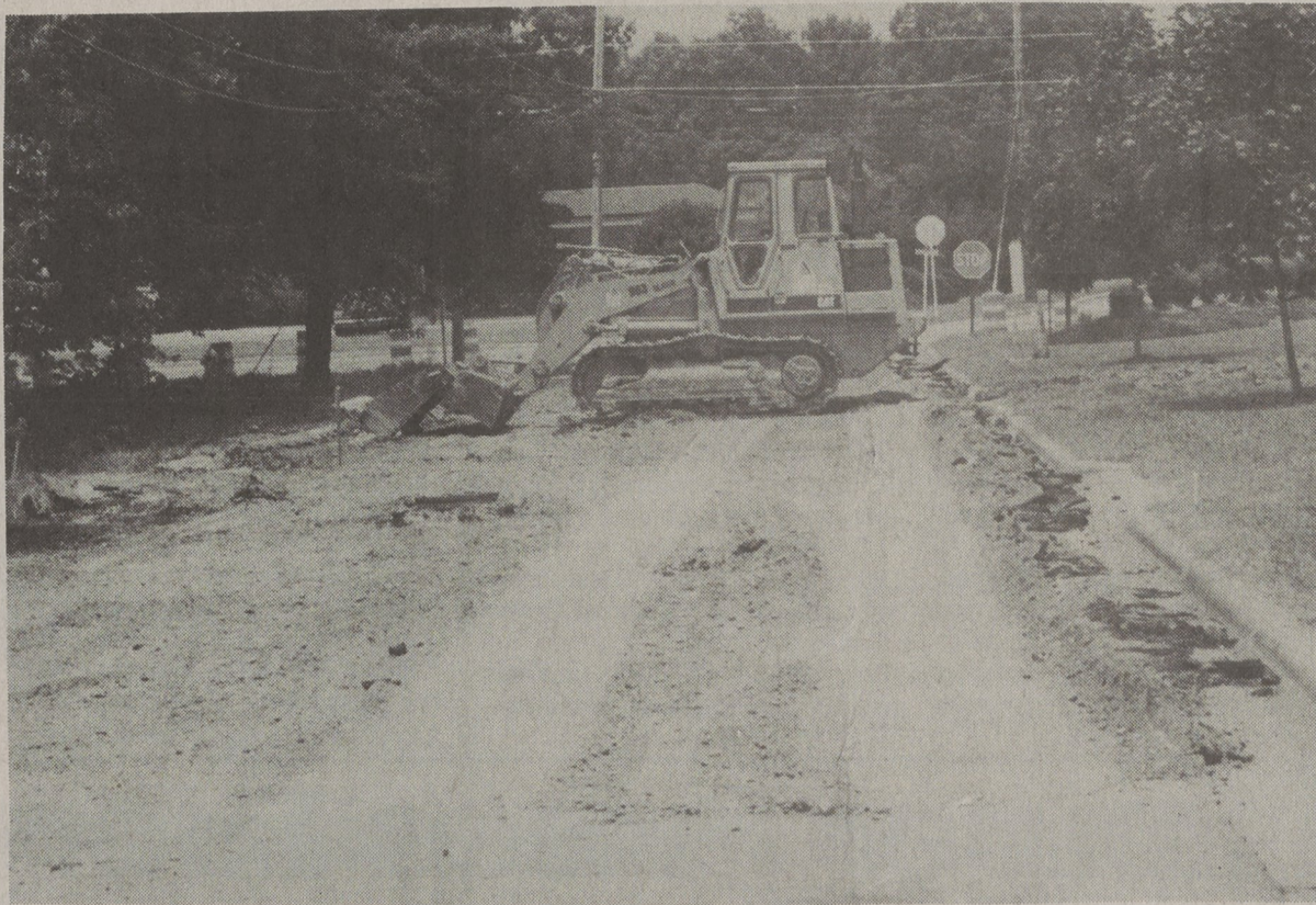
City crews are realigning South Sims Street in front of Home Federal Savings Bank. The street has been widened for a turn lane and city officials are hoping that the state will put up a stoplight.
