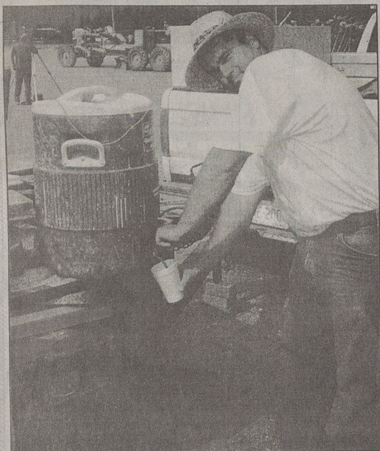
Alan Wilson stops to get a drink during work at the new mini-mall on Shelby Road in Kings Mountain. Temperatures approaching one hundred degrees had Wilson and his companions taking frequent breaks to stay cool.
