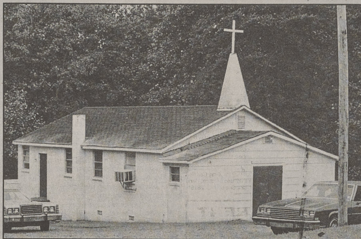
Open Door Mission Church, 309 Hillway Drive, Kings Mountain
