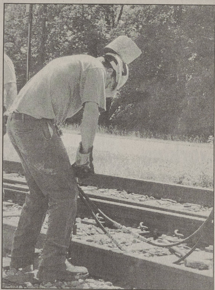
BEN LEDBETTER / THE HERALD Wayne Easley works with a jackhammer to break gravel at the railroad in Grover.
