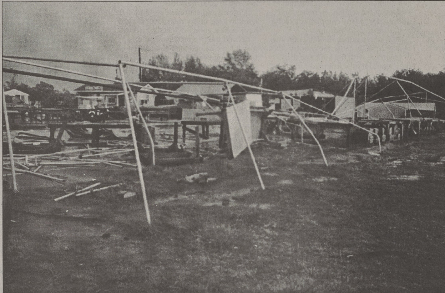
Betty Jones contributed this picture of some of the damage done by the thunderstorm and heavy winds Friday at the flea market across from Radio Station WKMT on Highway 161 north. Several trees were reported down in the area, including one that damaged a carport and house on Ridge Street, and there were a few brief power outages. Rain continued Monday and Tuesday and is expected to remain in the forecast through Friday.
