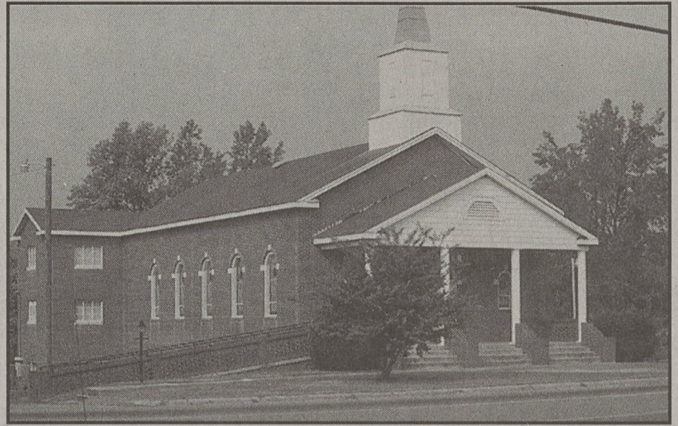
East Side Baptist Church - York Road - Kings Mountain
