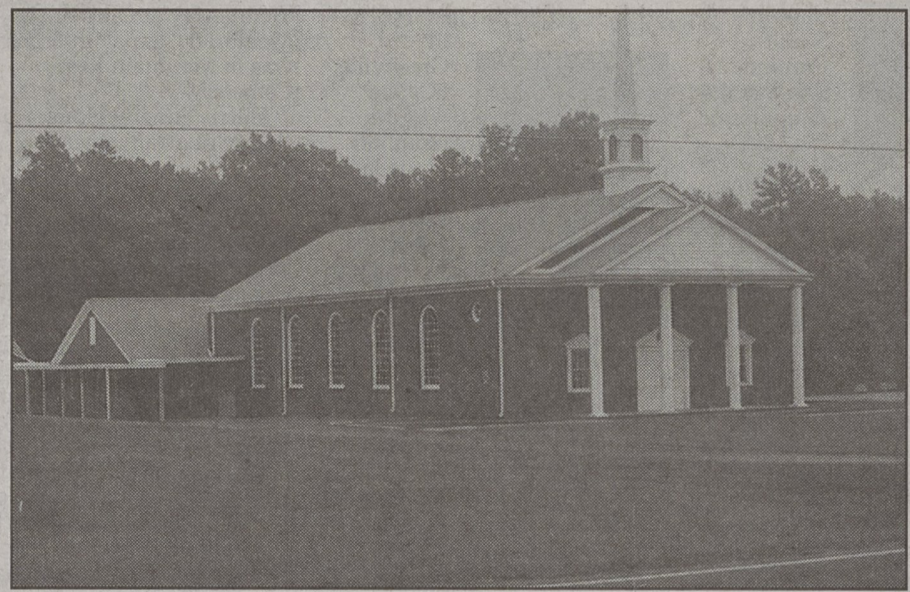
Oak View Baptist Church, 1517 York Rd., Kings Mountain, NC
