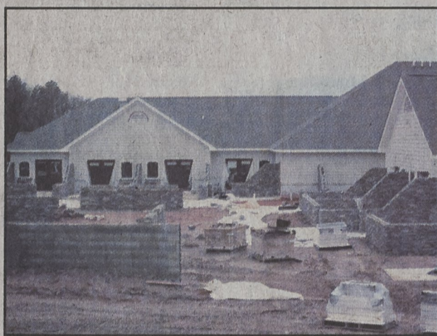
CONTRIBUTED PHOTO Work continues on the new KM Hospice House.
