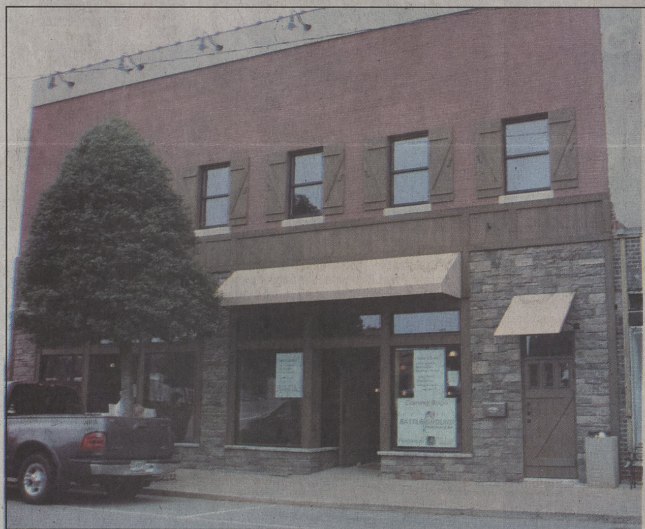
Fascade work for the new Battleground Steakhouse is complete. The restaurant is set to open for supper March, 23.
