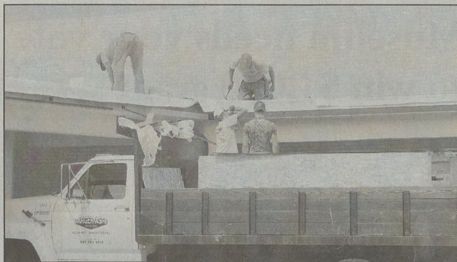
Workers finish some roof work at the high school last week.
